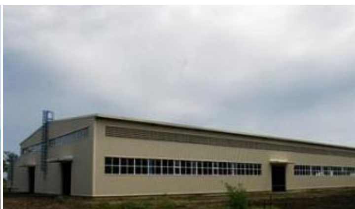
Completed Comprehensive warehouse
